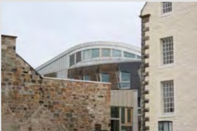
Metal roofing in an historic context—Canongate Stainless Steel roofing has been used on the Scottish Parliament
