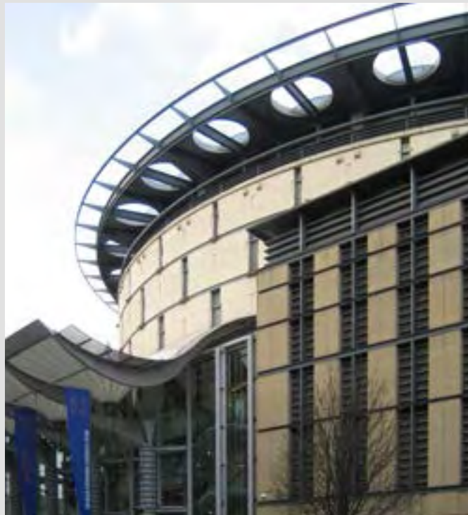
A mixture of cast stone & natural stone—Morrison St. Cast stone was used at high level on the drum shaped part of the building while natural stone was used at low level on the corners.
