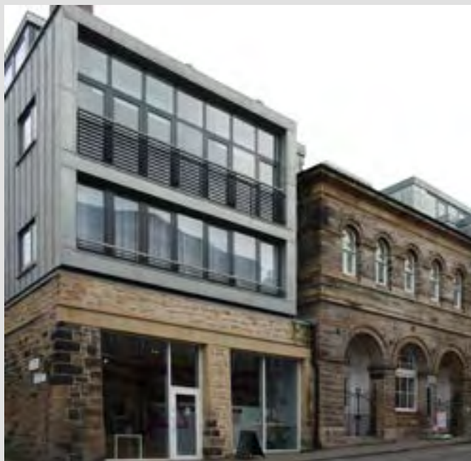
Using zinc to provide striking contrast—Infirmiry St. The zinc cladding combined with the modern building form provides a positive contemporary contrast to the historic former Infirmiry Street Baths building.
