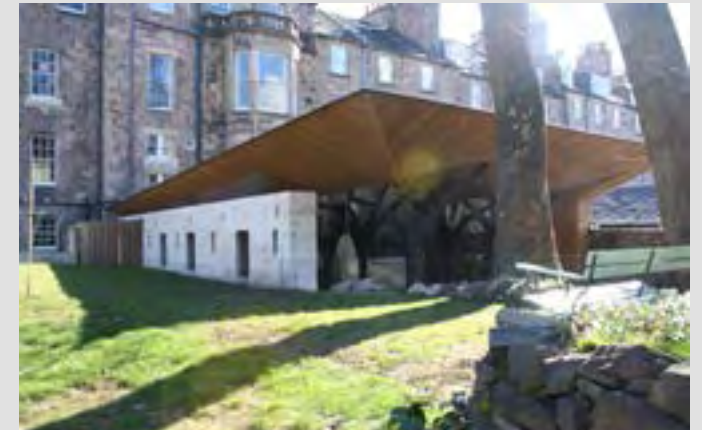
Frameless glazing—George Square Lane Glazing is used to create the effect of a floating roof on this religious building
