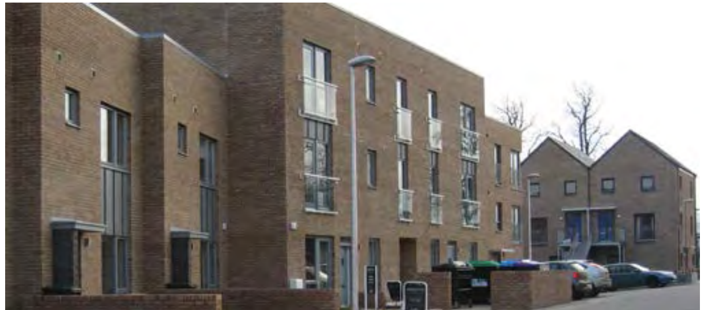
Tenure blind housing at Gracemount—Fala Place
