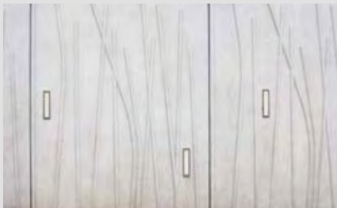
Concrete used sculpturally—Horse Wynd The sculptural potential of concrete is exploited in the Parliament wall with the patterned surface and integration of lights
