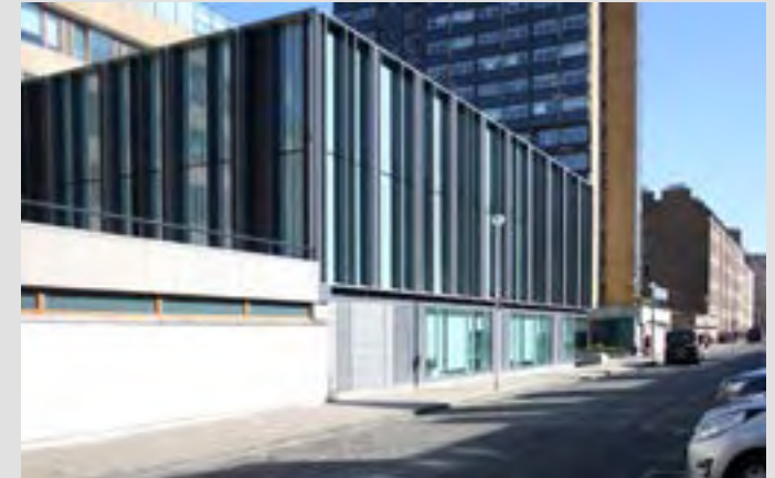
Curtain Walling—Beccleuch Place The potential offered by glazing systems with variations in the window widths, patterning of the glass and mullion depths is fully taken advantage of here.
