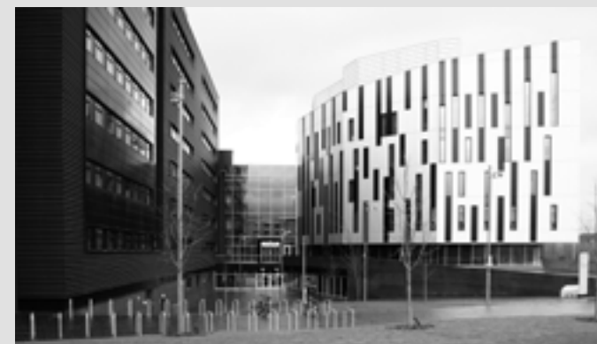
High quality detailing—Sighthill Court Construction of a sample panel and approval were required by condition in order to ensure the design intent of high quality finish was executed.
